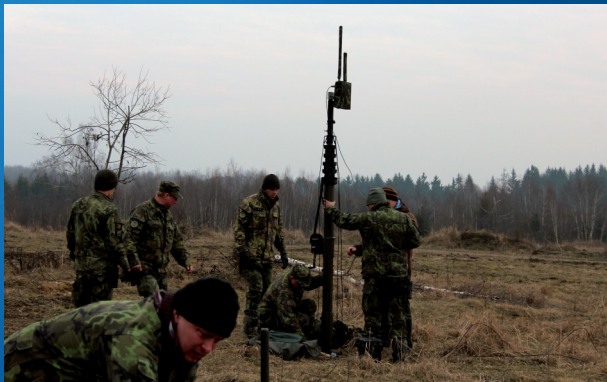
Installation of communication network
